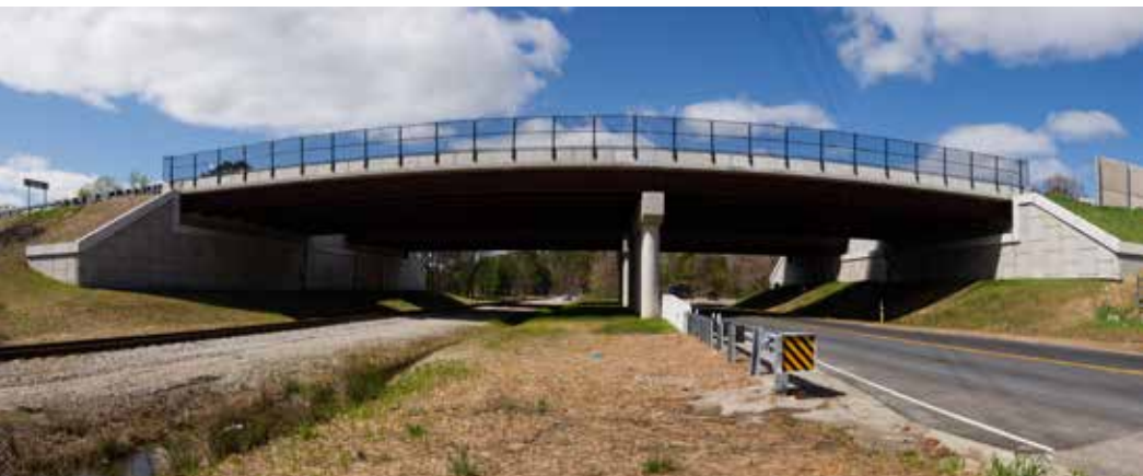
The team designed bridges and roadway approach grades over Industrial Park Drive and CSX Railroad that addressed soil settlement challenges, ultimately providing two new, two-span bridges in lieu of widening and repairing the existing three-span bridges.
