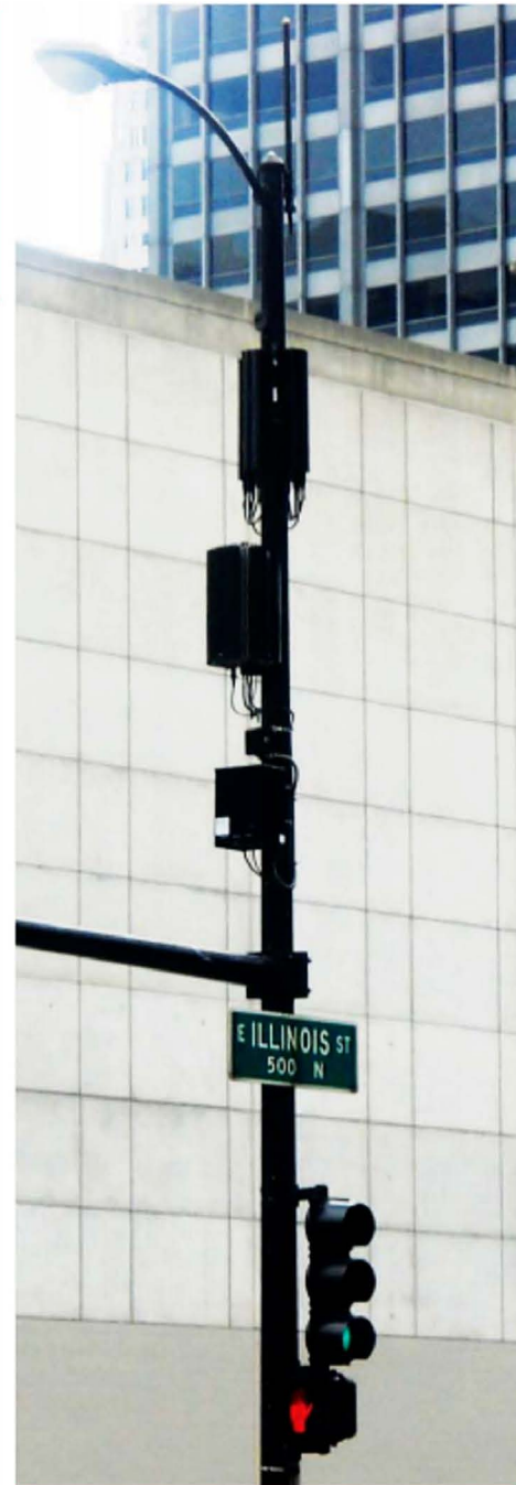
A standard option involves mounting antennas and equipment boxes on a light pole. Photo courtesy of Dewberry
